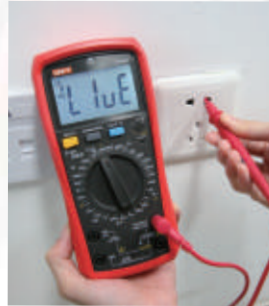
Live and nature wires identification
